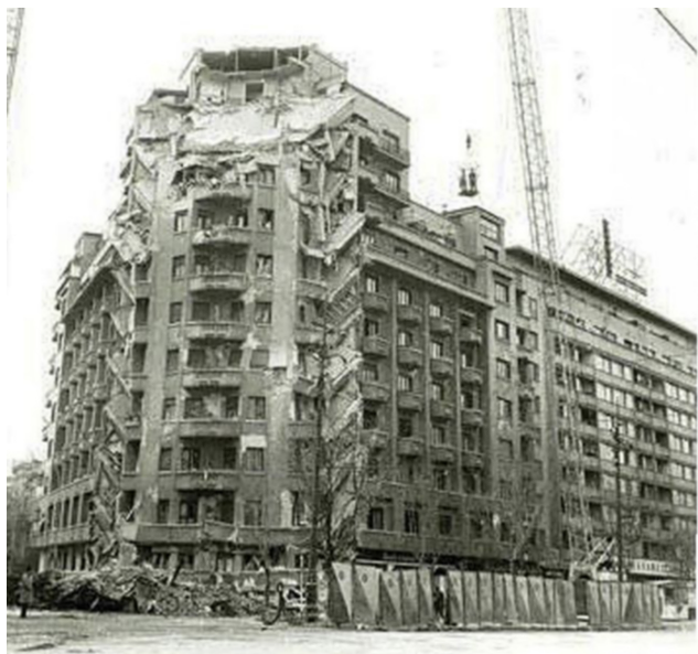
Figure 7. Wilson block of flats after earthquake (1977). Source: courtesy of Rezistența urbană (Urban resistance).
